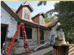
A combination of fiber cement and vinyl were used for the new siding.
