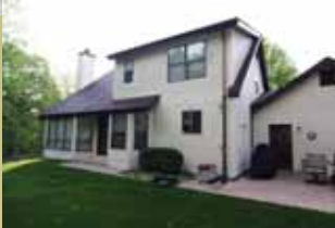
A combination of fiber cement and vinyl were used for the new siding.
