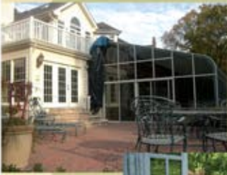
Signs of water damage appeared on the deck and pool house.
