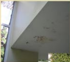
The peeling finish on the drywall suggested water damage which was confirmed as shown below.
