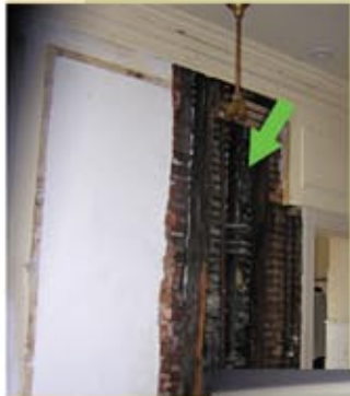
Pipes from roof to basement were removed.
